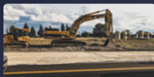
The construction site
